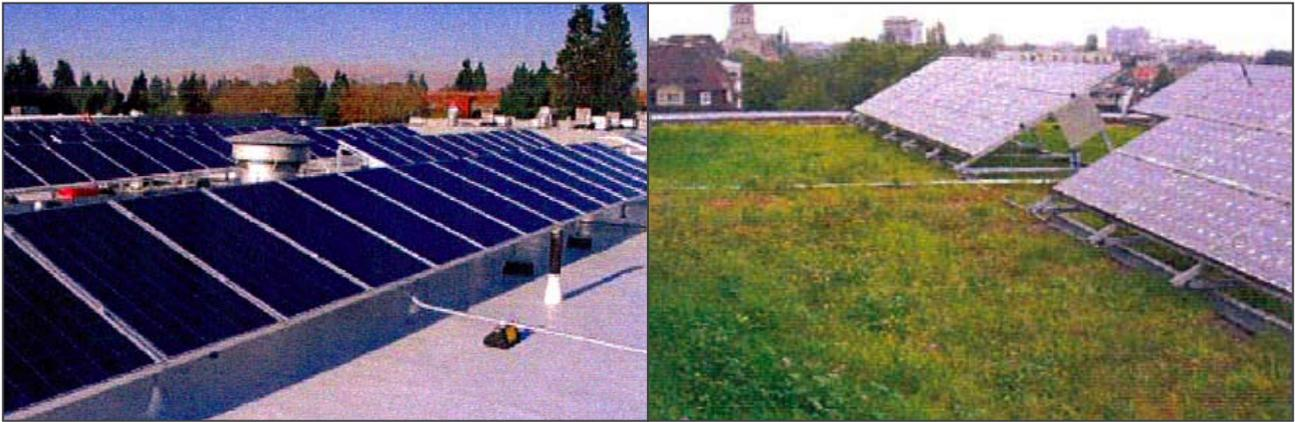
If we bring these two pictures together, it's fairly obvious how hot the uncovered roof can be and it is easy to appreciate how a Green Roof conditions the air and improves the efficiency of solar energy collection panels.
