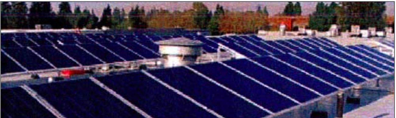
Gregg et al. while researching PV efficiencies for United Solar Ovonix LLC, found the performance of photovoltaic panels is lowered by 0.5%/°C above or below 25°C . Therefore at 60°C the efficiency is reduced by 17.5% affecting the payback period and economic viability of PVs.
