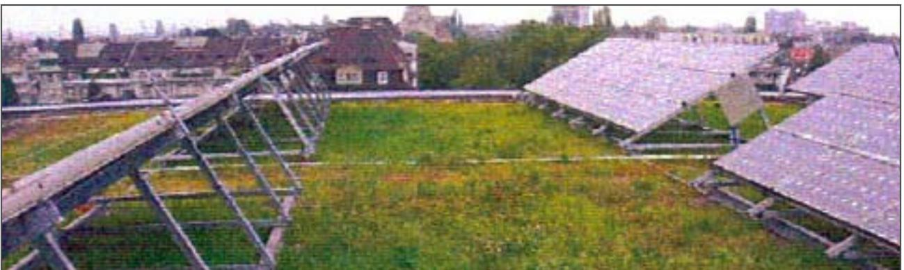
However, the use of a Green Roof maintains the ambient temperature at roof at about 25°C allowing the PVs to work at optimum efficiency
